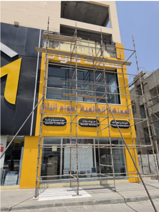
Sign preparation and on-site installation.
