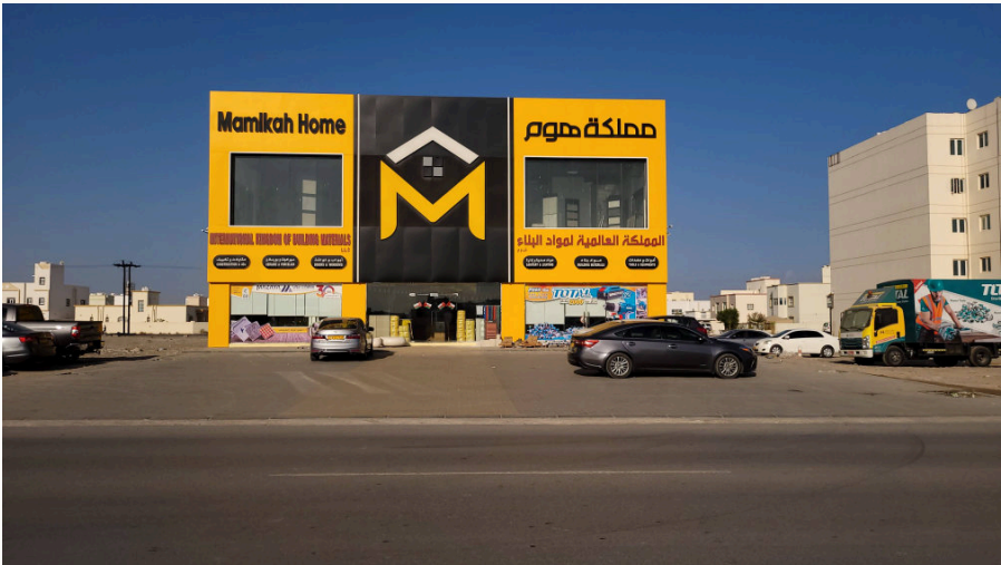
The facade after its signage and branding were fitted.
